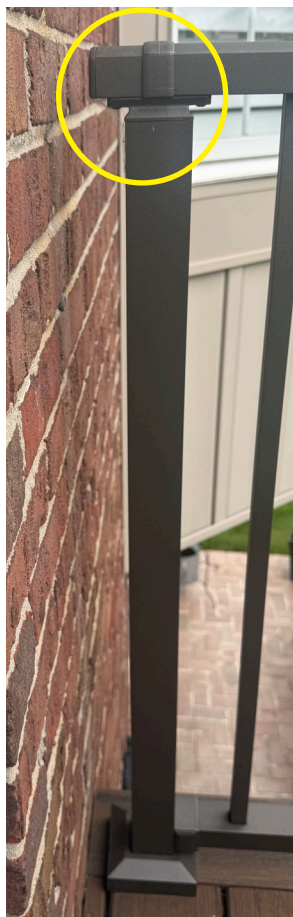
Railing does not touch building, no post cap, railing end cap
