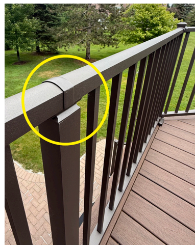
Level Crossover eliminates post caps on deck railing other than diagonal section
