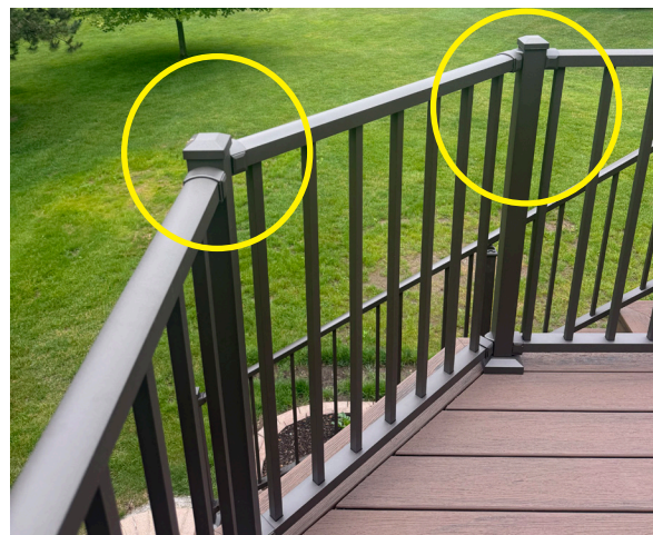
Post cap either side of diagonal section of railing (4 total)
